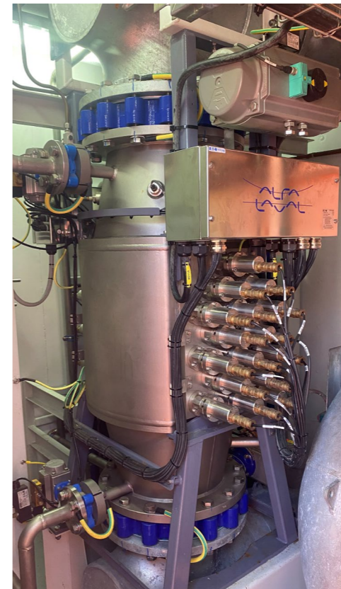
Ballast water treatment system on the Algoluna
